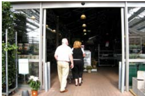
Duiven: customers witness the transformation, right from the start of the work.
